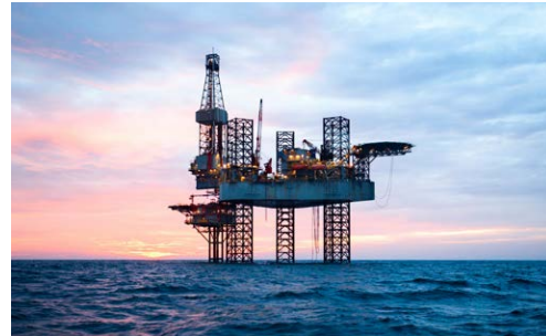
ENERGY, OIL & GAS
