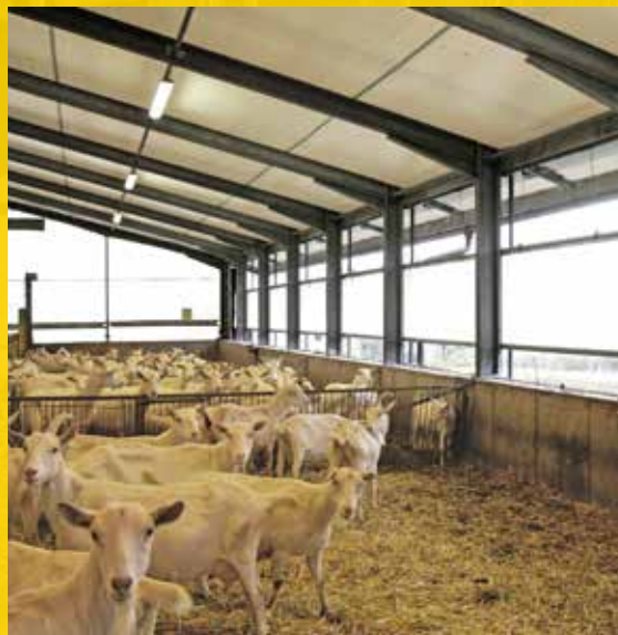
Animal welfare goat house in textile construction method with curtains in shading position
