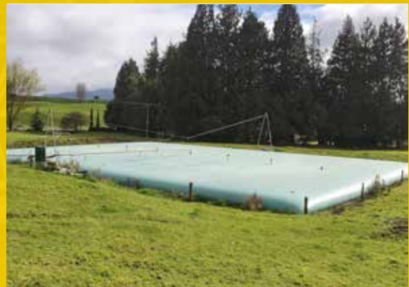
Waste water tank
