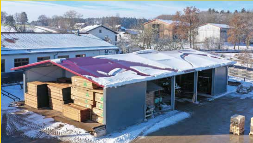
MACHINE HALL WITH CANOPY
