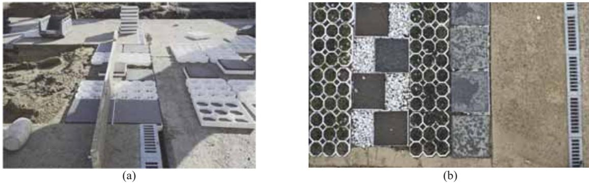
**Fig. 7.** Area Testing Scenario 3 (PMopenlab, R.ed.el Lab., 2018, Reggio Cal., Italy) (a) represent the implementation of recycled and printed components, (b) the final construction already in function of the green parking unit.
