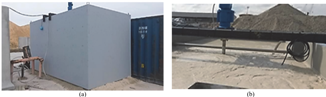
Fig. 1. Homogenization facility used during pilot testing: (a) storage and homogenization tank for collecting runoff water from clay heaps; (b) mixing process of the effluent to ensure uniform homogenization prior to treatment in the reactor
