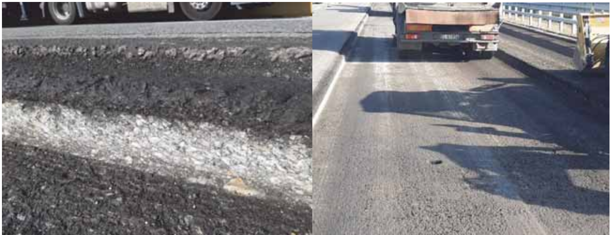
Fig. 2. Exiting pavement detail after the milling operation
