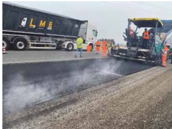
Fig. 3. Paving stage of GPC modified AC
