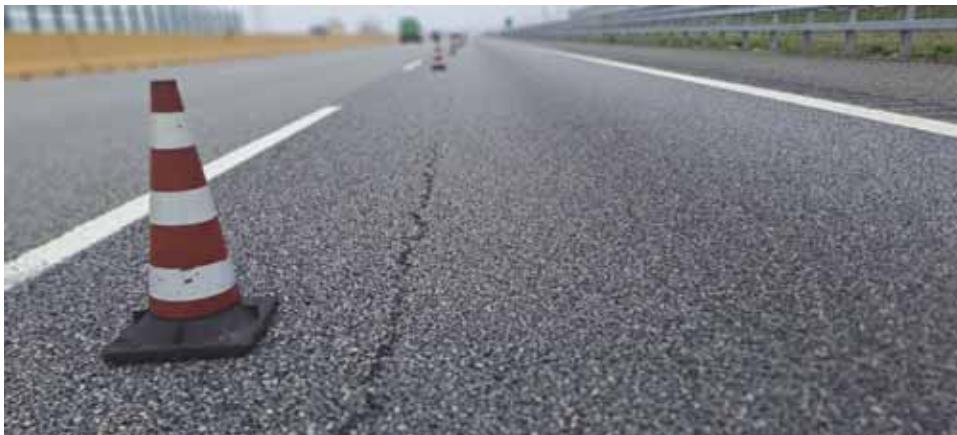
Fig. 12. Existing pavement monitoring (detail a)
