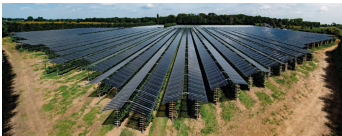
Figure 4-2 Light transmission achieved using transparent panels application. SolarPower Europe, 2020
